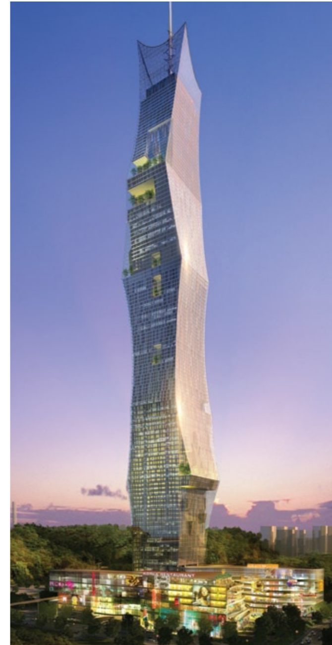
Seoul Tower Concept, Seoul, designed by Gensler A high-amenity, super-tall mixed-use tower, overlooking the Han River, designed to accommodate a vertical lifestyle.
